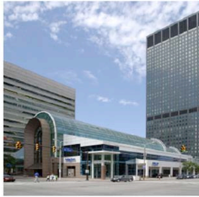
Dollar Bank/ Renovation of the Galleria at Erievue Cleveland, OH First Place, Retail Renovation, VM+SD National Design Competition City of Cleveland Redevelopment Project of the Year IIDA Cleveland Design Award
